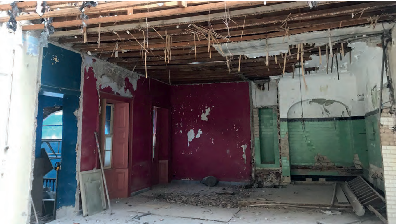
Further demolition and roof removal
